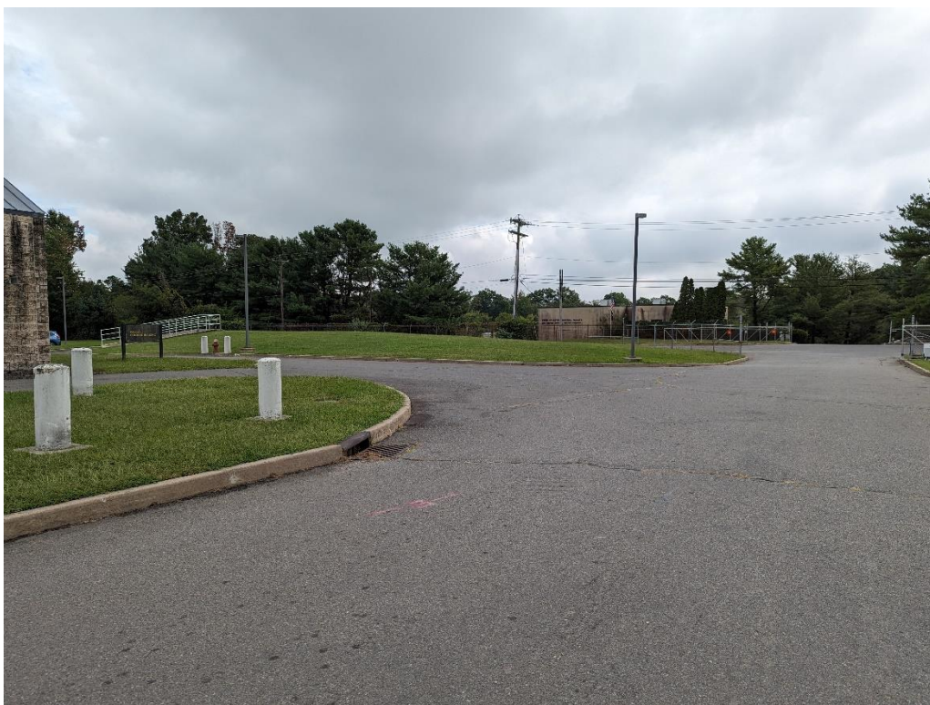
Photo 15: View facing east toward Millstone Road in existing facility. East Windsor, NJ, 9/11/23.
