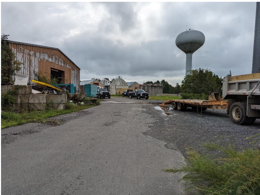
Photo 14: View facing east in existing facility. East Windsor, NJ, 9/11/23.
