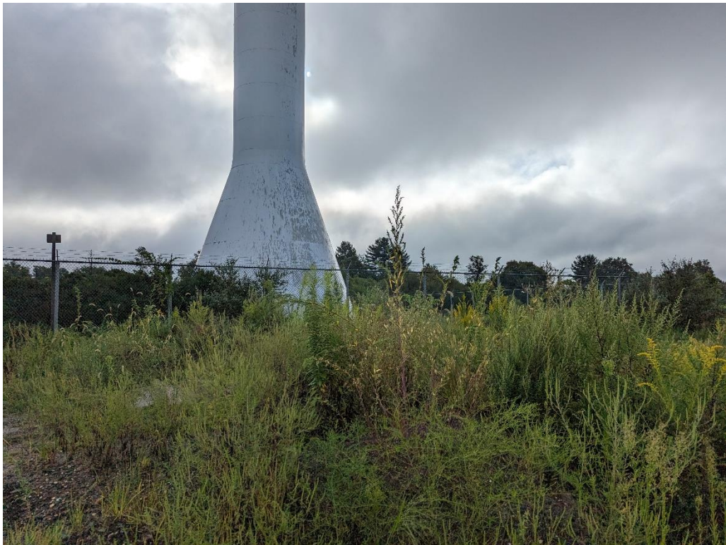
Photo 3: View facing north toward existing water tower. East Windsor, NJ, 9/11/23.
